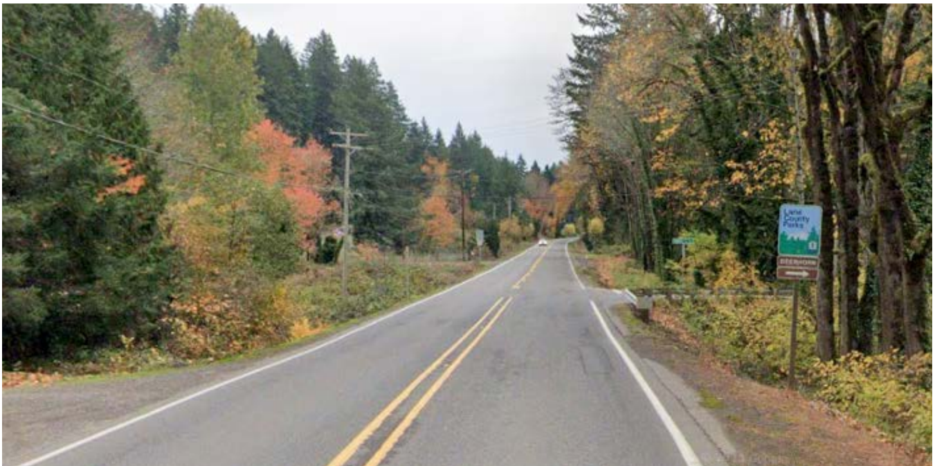
FIGURE 6. OR 126 EAST AT HOLDEN CREEK LANE (WEST), LOOKING EAST
