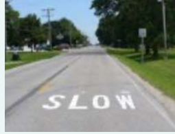
“SLOW” PAVEMENT MARKINGS
