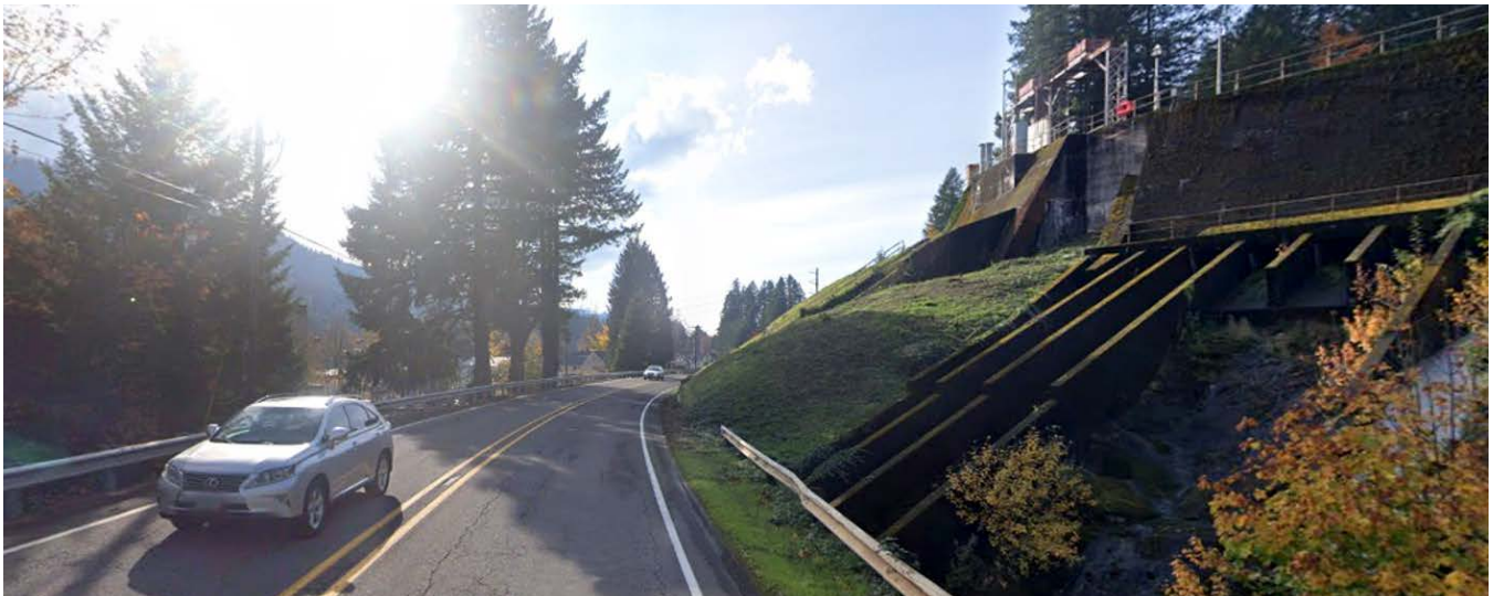
FIGURE 8. OR 126 EAST AT LEABURG DAM SPILLWAY, LOOKING WEST
