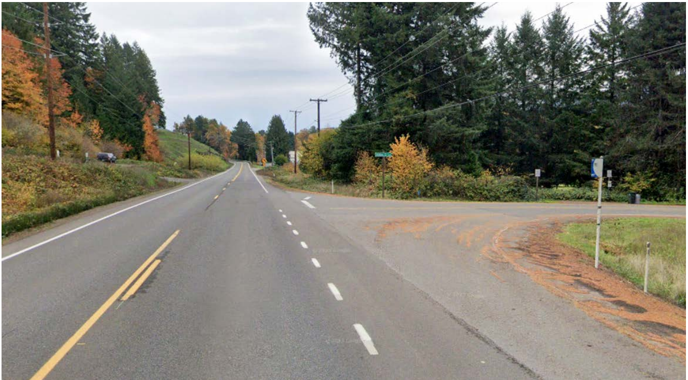
FIGURE 7. OR 126 EAST AT HOLDEN CREEK LANE (EAST), LOOKING EAST
